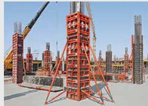
Column Formwork
