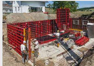
Wall Formwork
