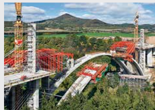
Bridge Formwork
